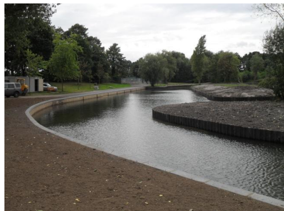
After including realigning and renewing masonry
