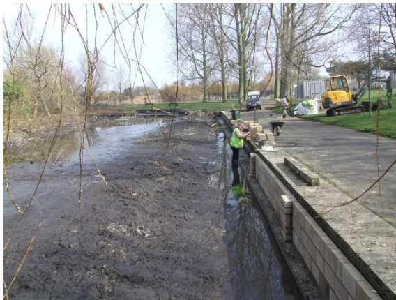
Re-facing existing masonry wall
