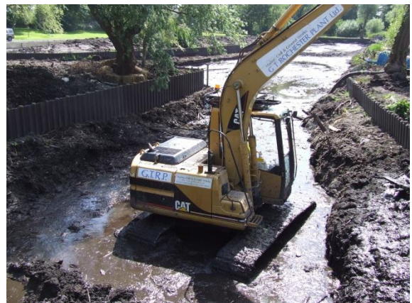
Dredging at the deepest point of the lake
